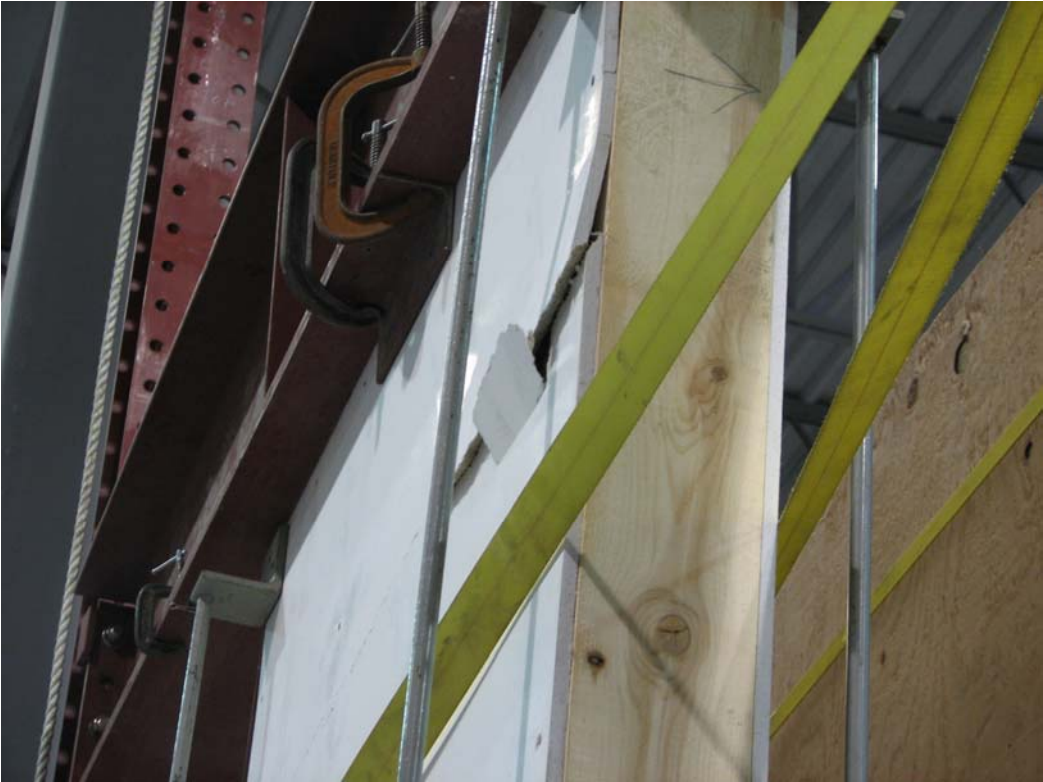
Wood panel specimen 3 for axial load, product sheathing failure
