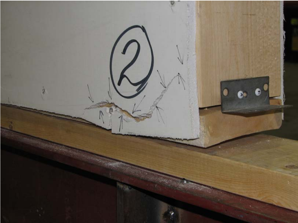
Wood panel specimen 1 for racking load, product failure at location 2
