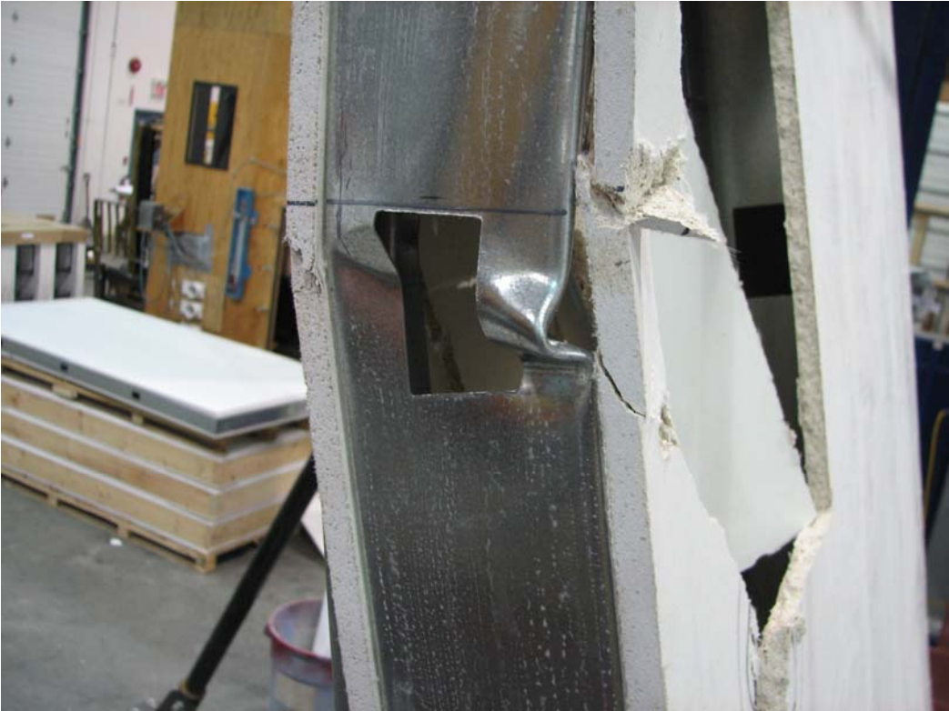
Metal panel specimen 1 for axial load, product failure due to buckling
