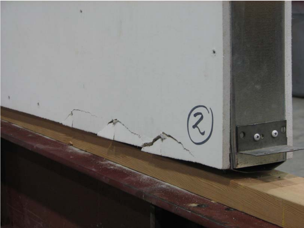
Steel panel specimen 1 for racking load, product failure at location 2
